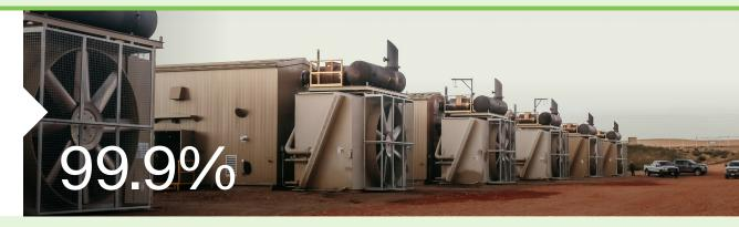
Crusoe's DFM™ technology converts the natural gas captured at oil wells and converts it into electricity by leveraging a stoichiometric combustion process, which allows reaching a 99.9% methane destruction efficiency.
